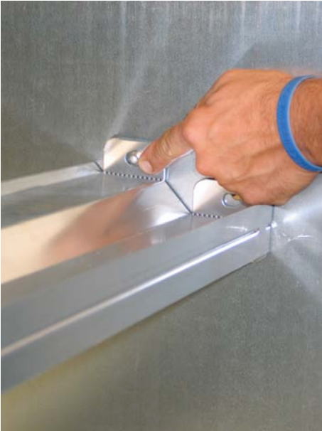
Tighten the TBEI M8x16 screws
