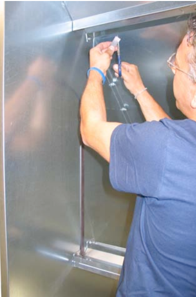
Tighten the TBEI M8x16 screws
